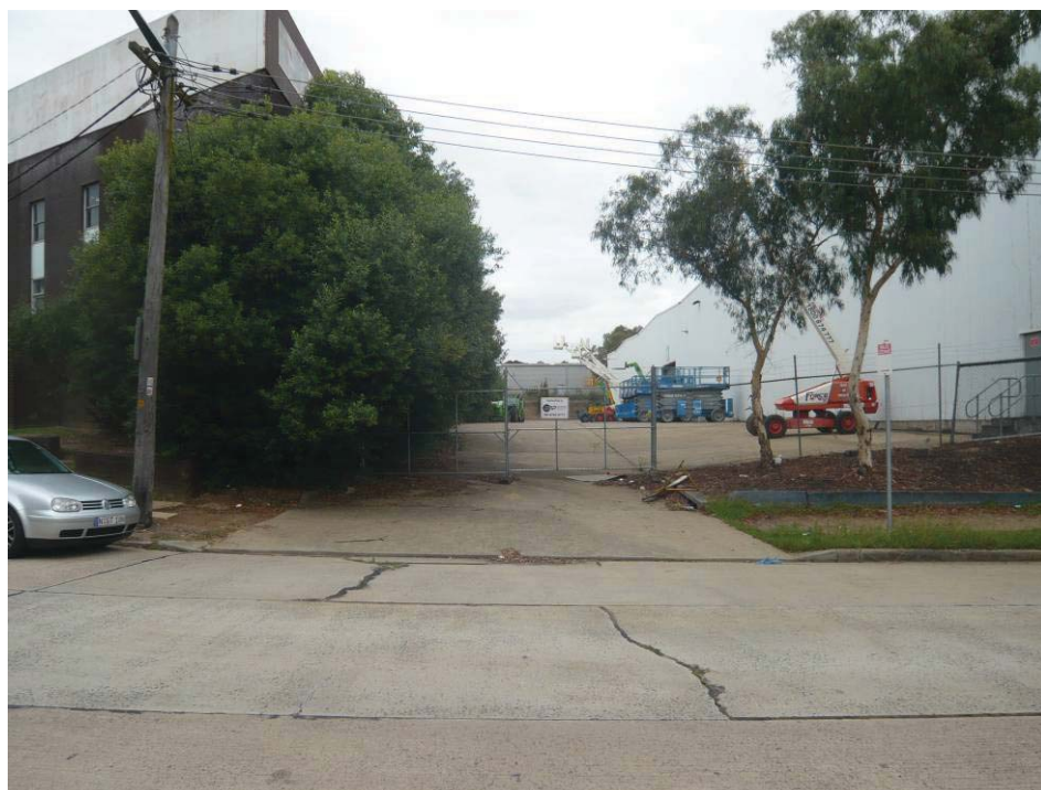
View east across Uhrig Road towards the access situated in the northwest corner of the site.
